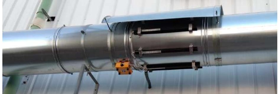
**Static elimination system for piping -
